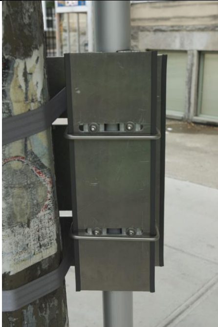
C: Bracket Installed Using Mounting Hardware To Secure Pole
