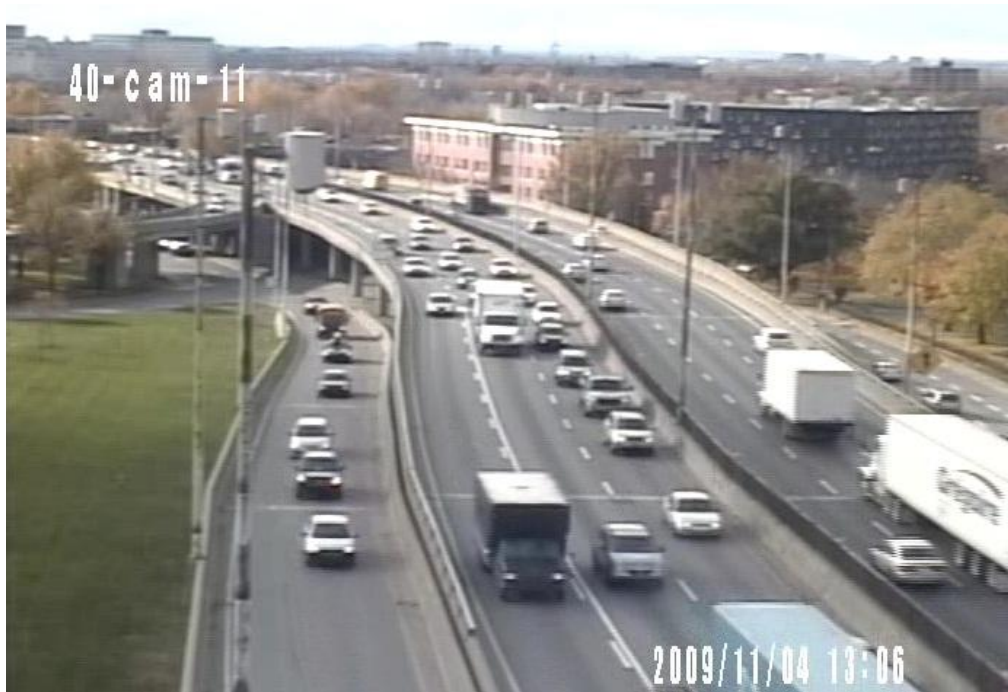
Figure 7 – Autoroute 40 “Autoroute métropolitaine” eastbound, entrance 73, “Christophe-Colomb”, view from Cam40-11-westbound, with LCGV1 treatment. Horizontal and vertical curves can affect user visibility, particularly for entrance merging manoeuvres.
